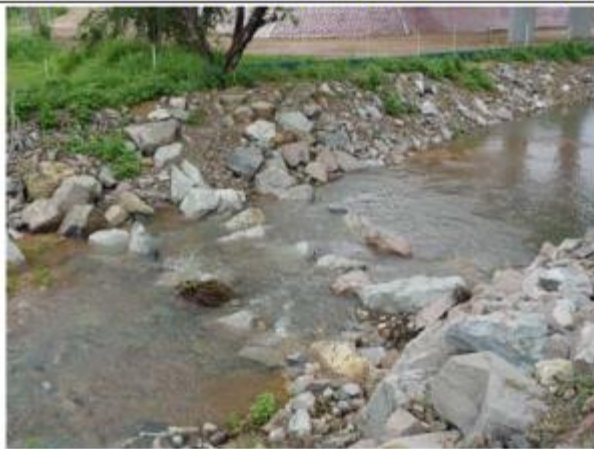
Douglas Arterial Project rock ramp fishway within open channel diversion drain at bridge site (25/01/05)
